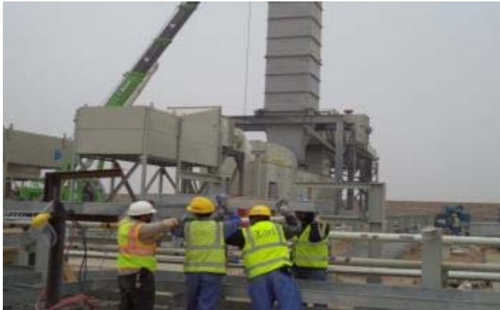
Cable Ladder Work
