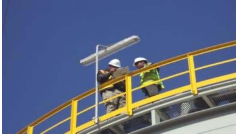
Light Fixture Installation
