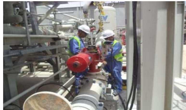
Installation of Instrument Devices
