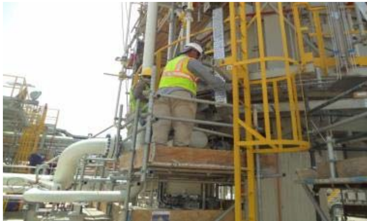
Installation of Tubing
